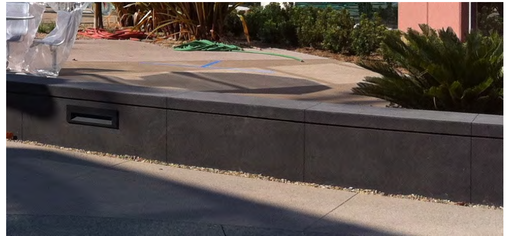
Cast-in-place concrete seat wall
