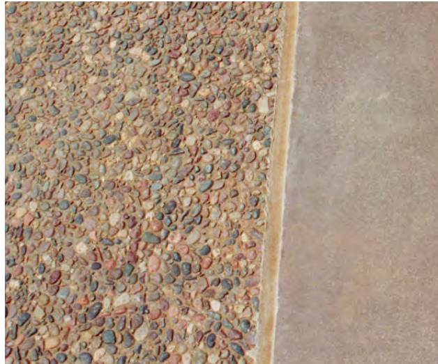
Hand seeded aggregate concrete paving
