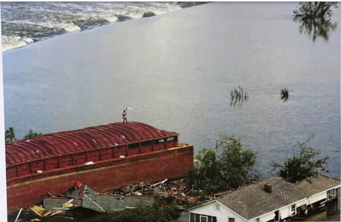
Floodwaters flow over a failed levee along the Inner Harbor Navigation Canal near downtown New Orleans following Hurricane Katrina, while a trapped resident waves a white flag for help. A major flaw of New Orleans's site is found in its low-lying land along Lake Pontchartrain and the Mississippi River. Massive flooding devastated the region after Hurricane Katrina struck in 2005.
