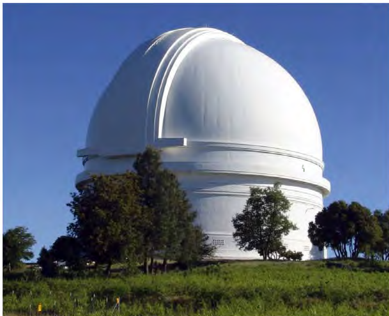
This building houses the Mount Palomar telescope. The dome opens when the telescope is being used.
