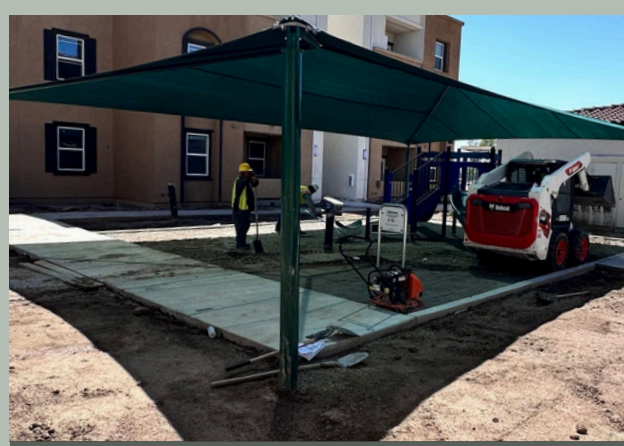
KOMPAN Shade, Grading and Preparation, PIP Playground Structure Installation
